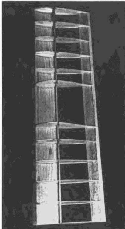
Wing with L.E. sheet, lower capstrips, and T.E. filler pieces installed.
