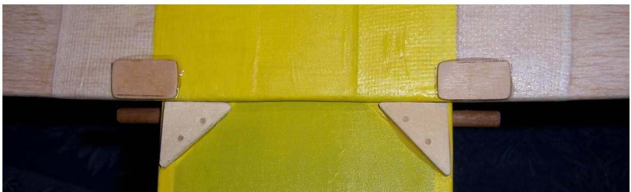
Ply plates for further wing band reinforcement and wing mount position epoxied in place.
