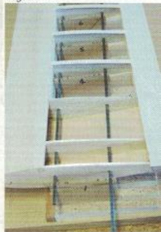
Below: Front and rear sheeting added. Note piano wire alignment
