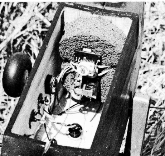
One-sided gas tube receiver in crash-proof installation. Plan gives details for the McNabb.
