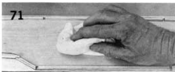
71. Rub down the plywood doubler thoroughly with a rag and continue doing it until the glue has completely set up. Full cure of 5 minute glue takes several hours or more so it is advisable to weight the doublers down for awhile for best results without any curling or warping.
