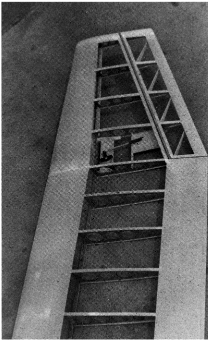
Completed wing section.
