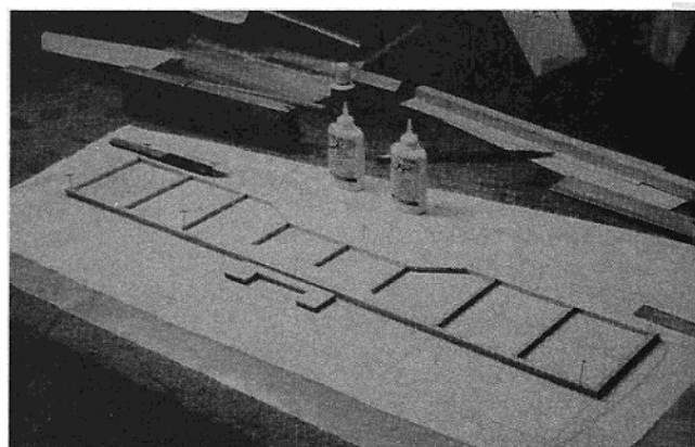
Stabilizer under construction. Ply elevator joiner in position.
