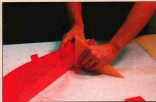
When installing the bulkheads, use a triangle (this one's cut from scrap wing material) to ensure squareness.
