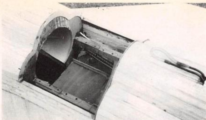
Access hatch and fuselage opening are lined with 1/32" plywood to help prevent deformation. Note cheater hole opening in bottom of inlet passage.
