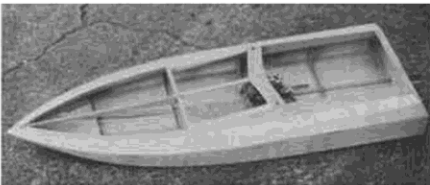
Top deck framework and hatch framework ready for sheeting.
