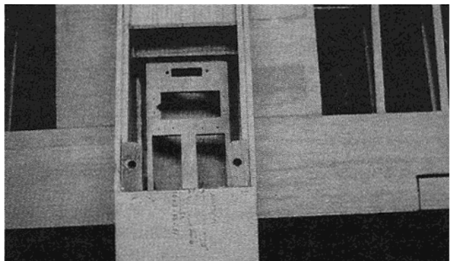
Maple blocks are drilled and tapped for wing mounting bolts.
