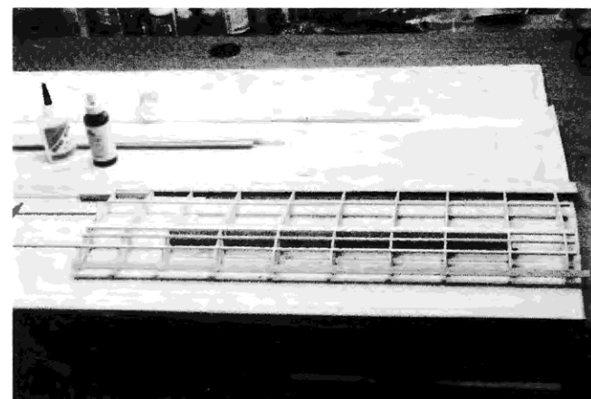
start adding the top spars, leading edge and top trailing edge sheet (above right). Note the shear webbing and the filler blocks in the center trailing edge.
